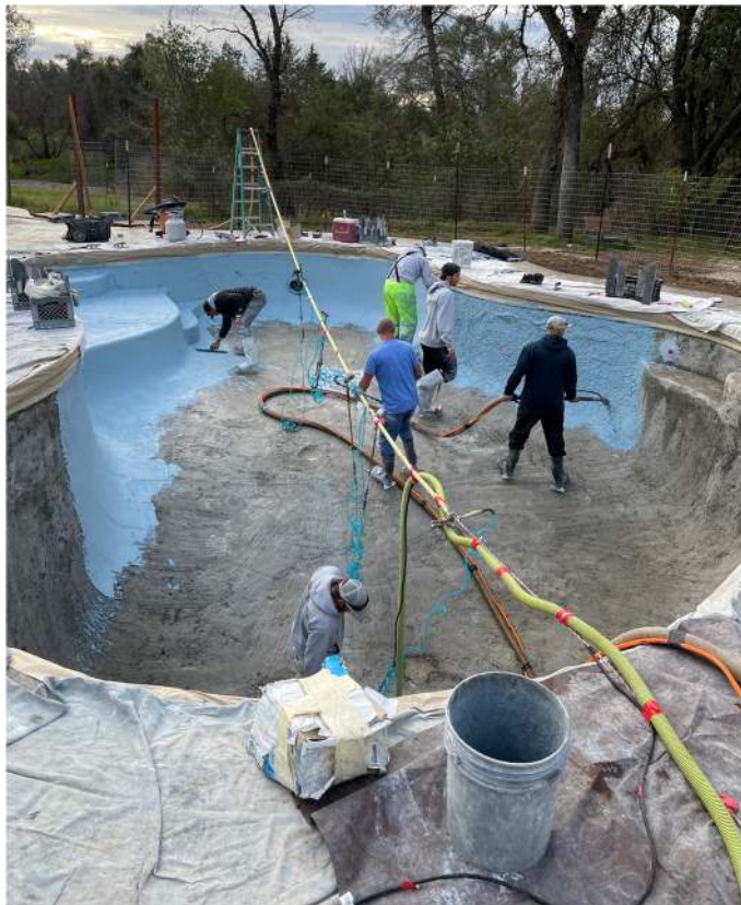
Figure 1. A typical US exposed aggregate, swimming pool finishing mix being applied.
