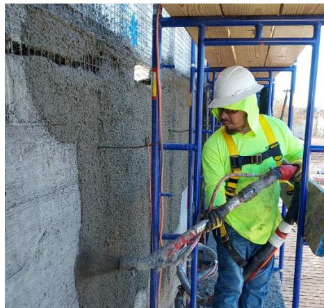
Figure 3. Shotcrete mix with EdenCrete® filling and fully encapsulating the wire mesh
