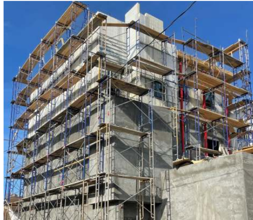
Figure 2. 4-storey SCIP residential home in Houston under construction and including EdenCrete®
