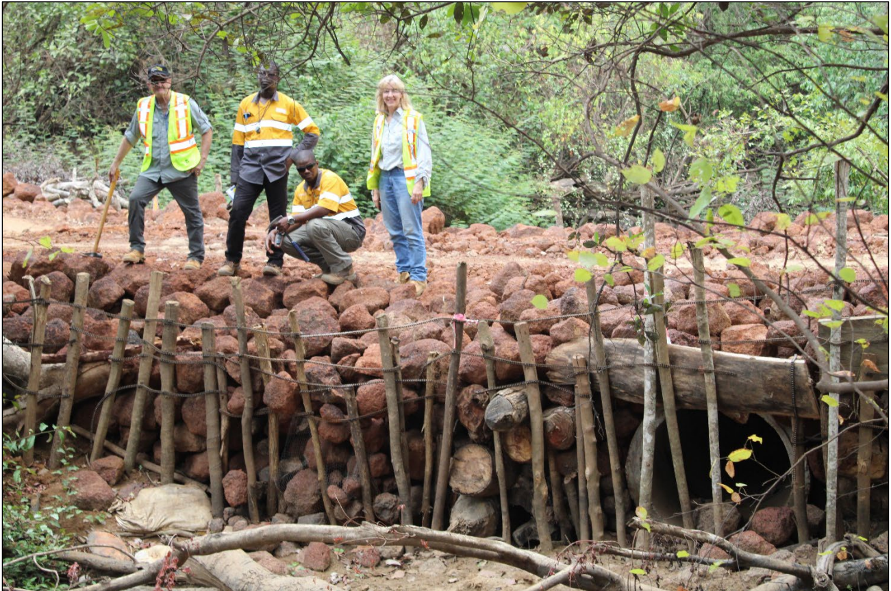
Figure 14: Traditional laterite bridge which provides access from Gogbala to Tchaga during the wet season
