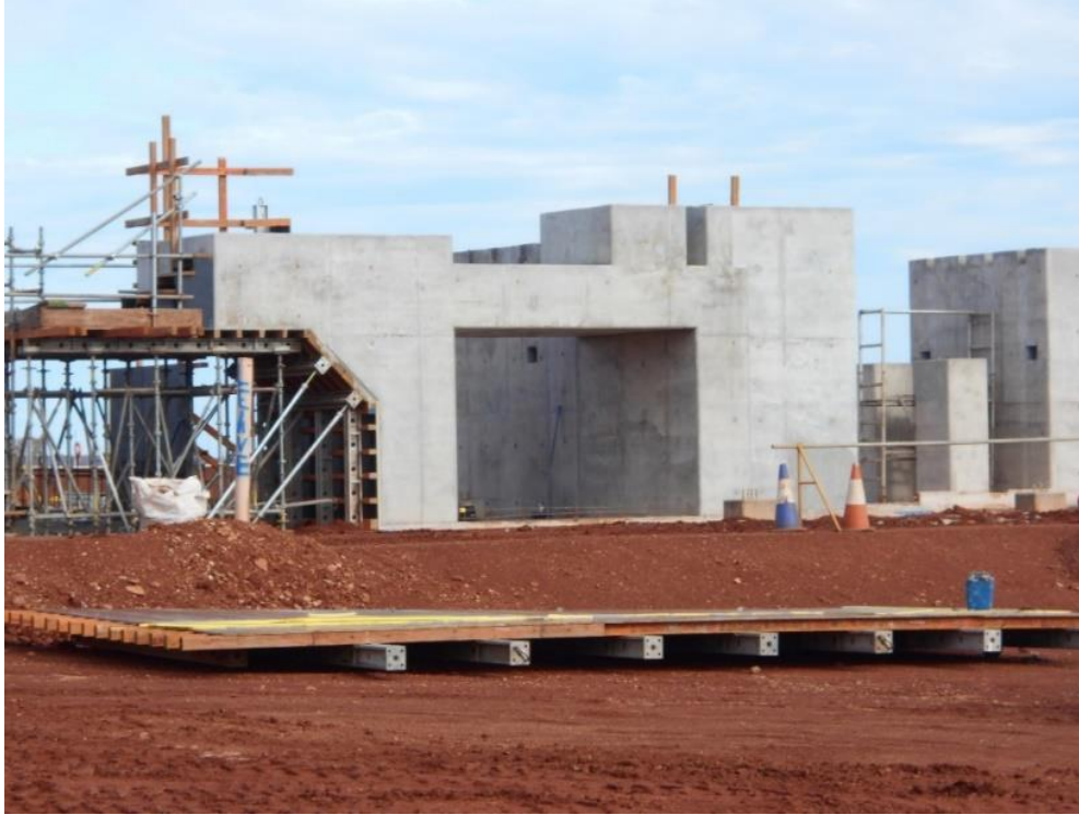
Figure 6. Grinding mill plinths.
