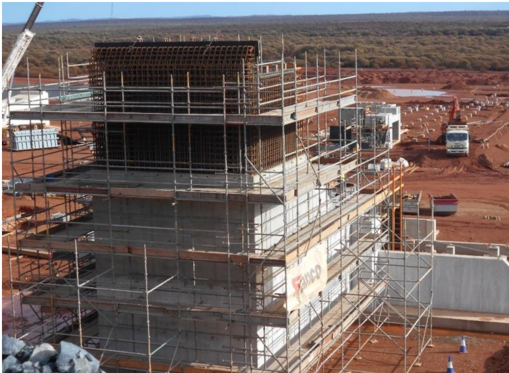
Figure 5. Crusher with formwork and rebar in place prior to third concrete lift (now complete).
