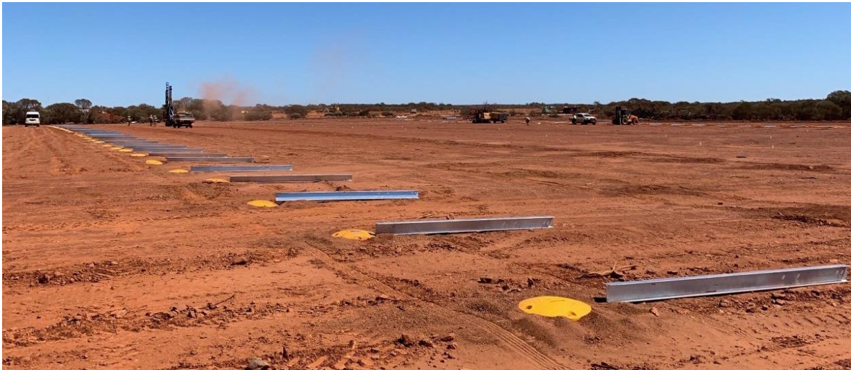
Figure 7. Post-hole drilling and solar panel supports.
