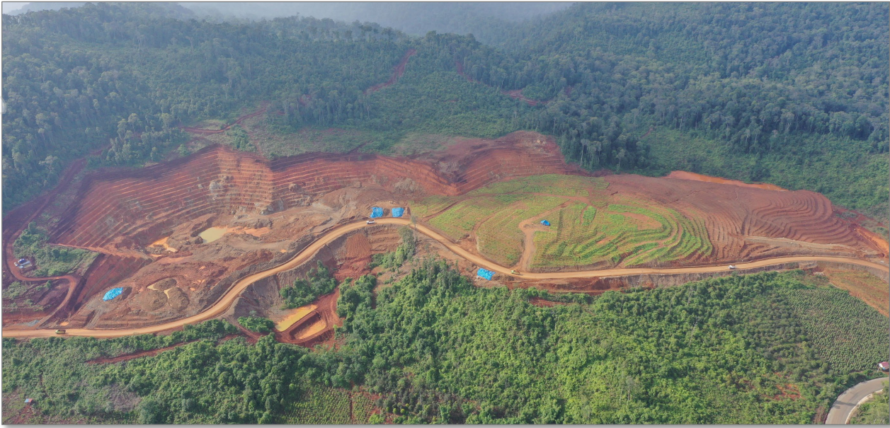
Central Pit rehabilitation has commenced
