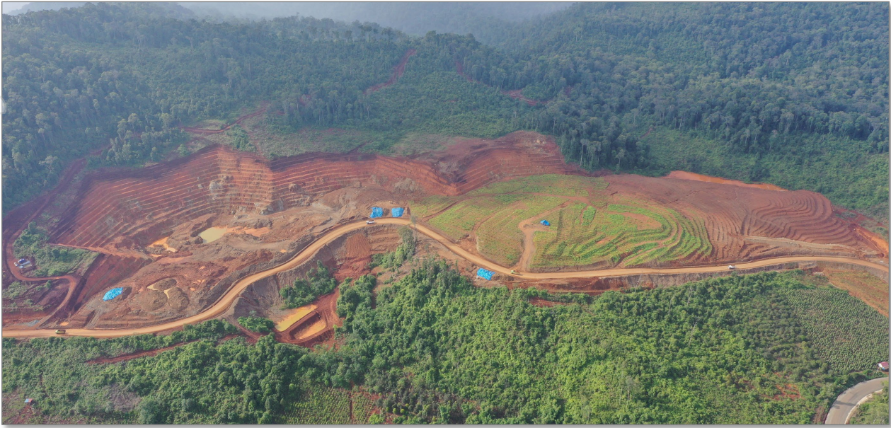
Central Pit rehabilitation has commenced
