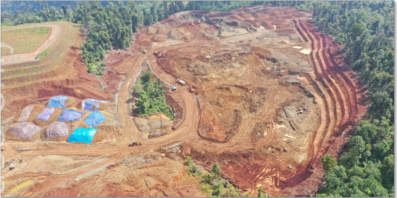
Bete Bete East pit extension
