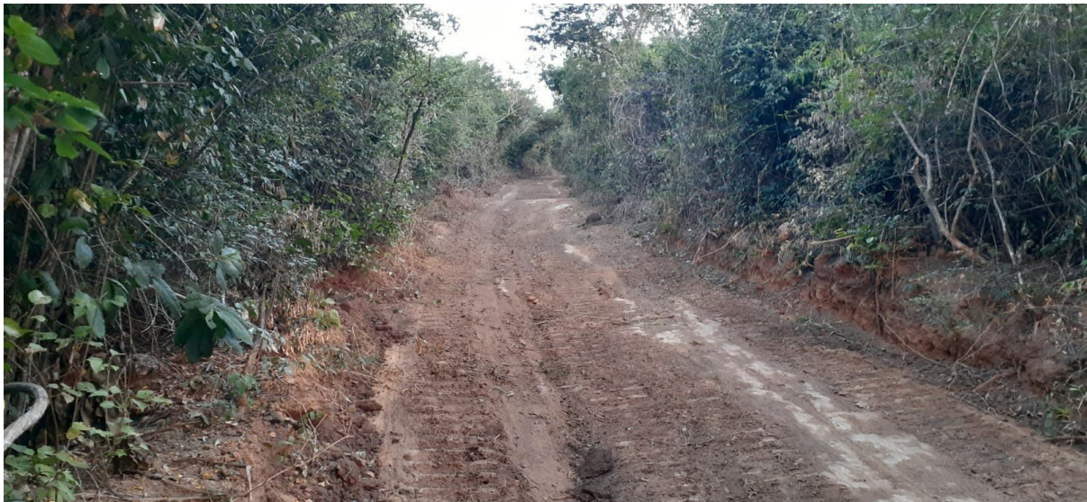
Figure 4: New site access track completed at the Monte Alto Prospect – Salinas Lithium Project, Brazil
