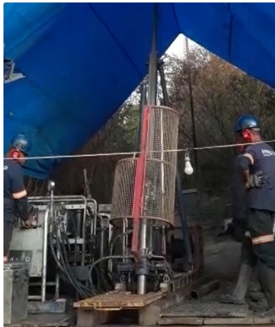
Figure 2: Diamond drilling at Salinas Lithium Project, Brazil
