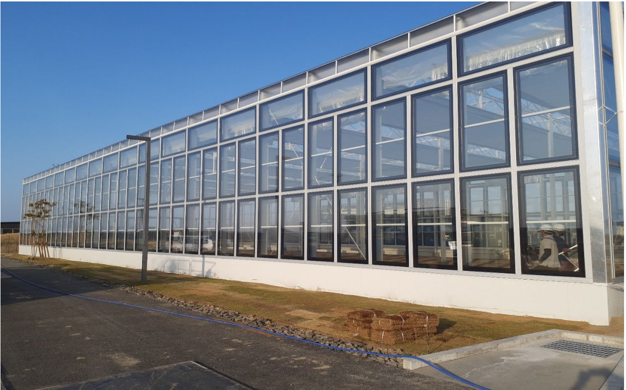
Completely glazed greenhouse at Aqua Ignis Sendai showing installed ClearVue PV IGU panels of custom dimension - 1.908m high x 0.95m wide around all sides of the greenhouse.
