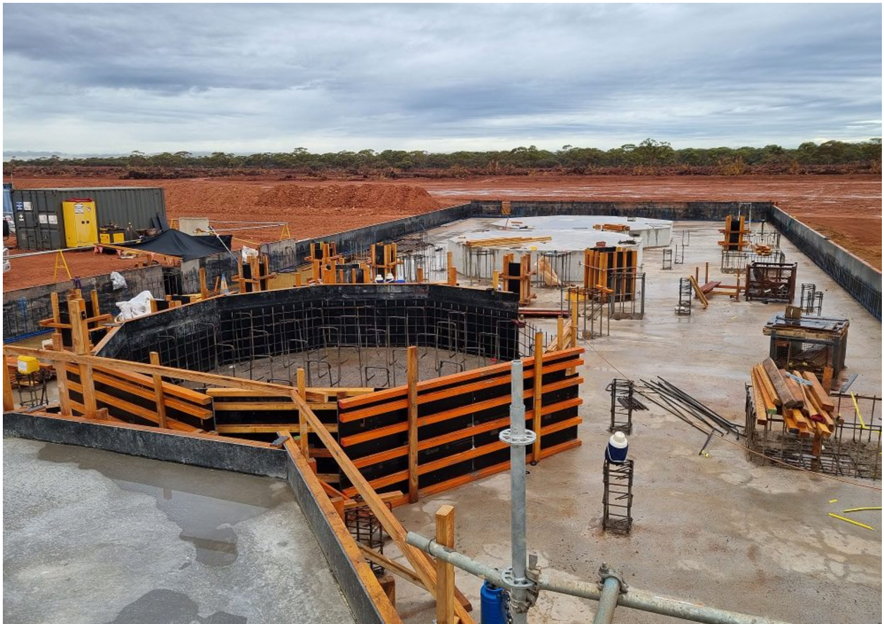
Soda ash area civils with floor and two tank supports completed
