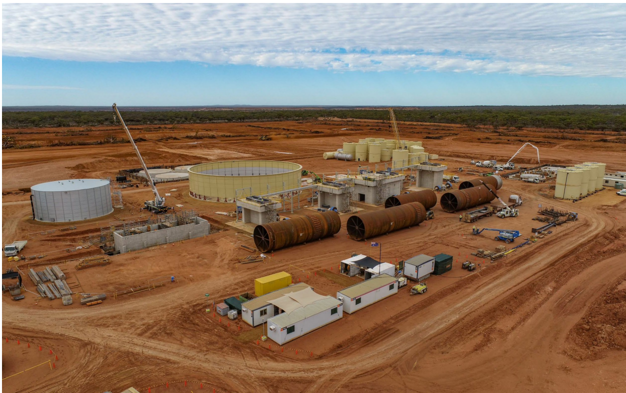
Aerial view of Kalgoorlie construction works, March 2022
