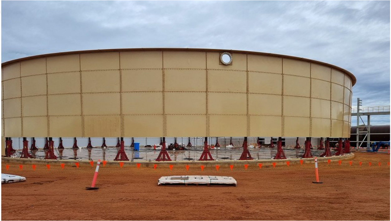
Raw water tank during construction of fifth level
