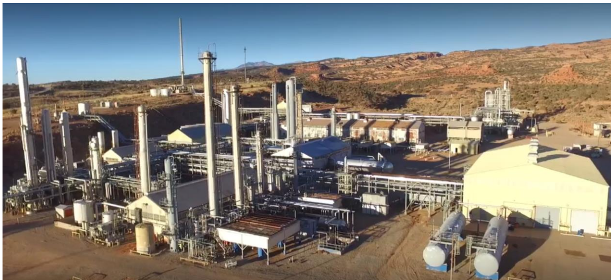
Figure 1 – Lisbon Valley Gas Plant
