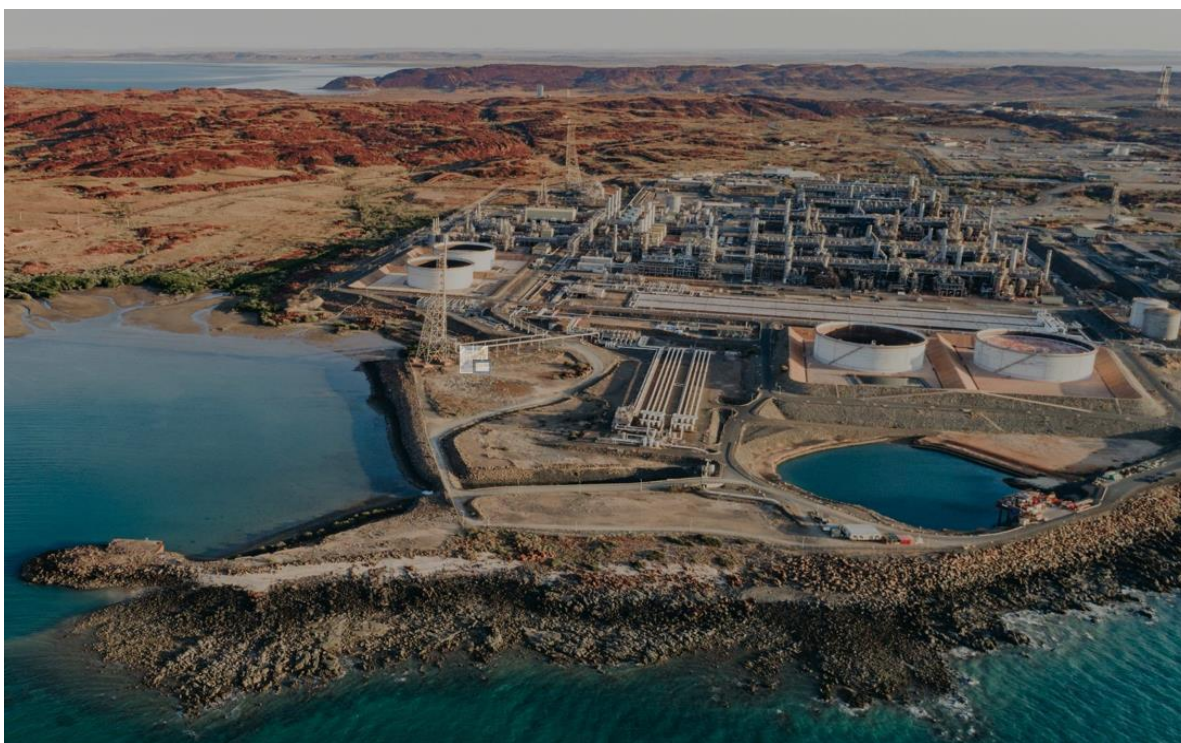
Figure 4.5: Karratha Gas Plant
