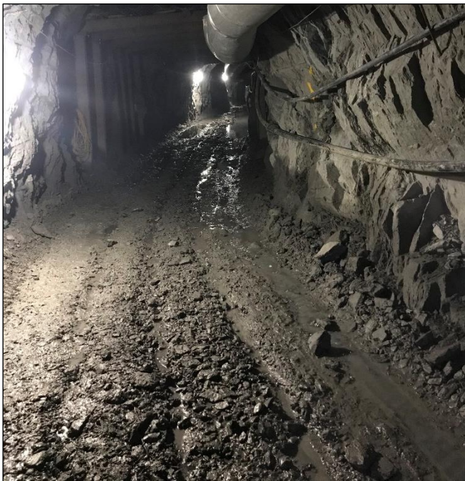
Figure 2 - In Progress Development Drive
