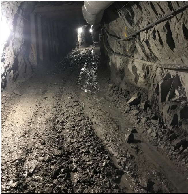
Figure 2 - In Progress Development Drive
