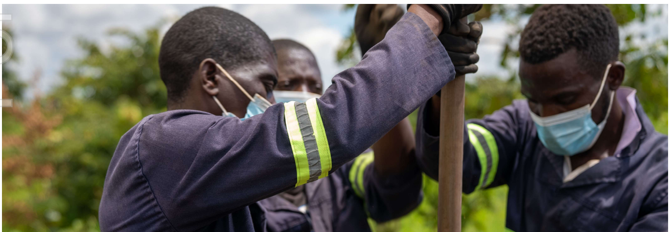
Figure 7: Hand-auger drilling at Kasiya
