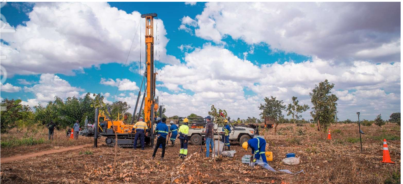
Figure 13: Core drilling in action at Kasiya
