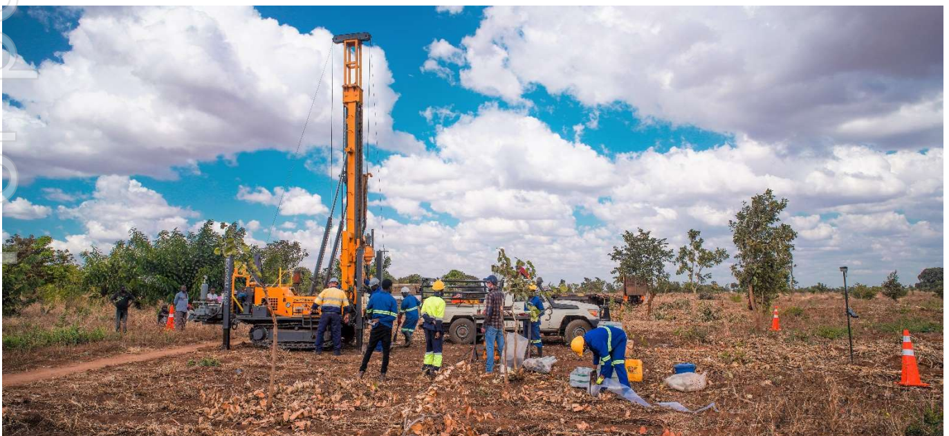
Figure 13: Core drilling in action at Kasiya
