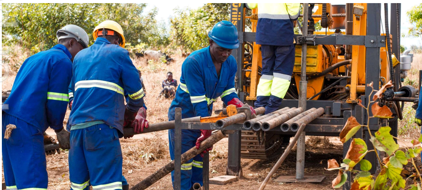
Figure 5: Core drilling at Kasiya
