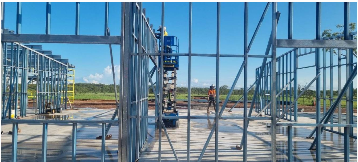
Figure 1. Steel wall framing of the Finnis site administration office complex
