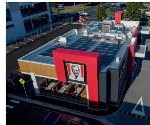
TAKANINI RESTAURANT SOLAR PANELS
