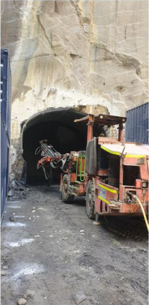
Figure 5 Komatsu MC51 commencing the portal for the ventilation drive (LHS) and jumbo installing the portal ground support (RHS)
