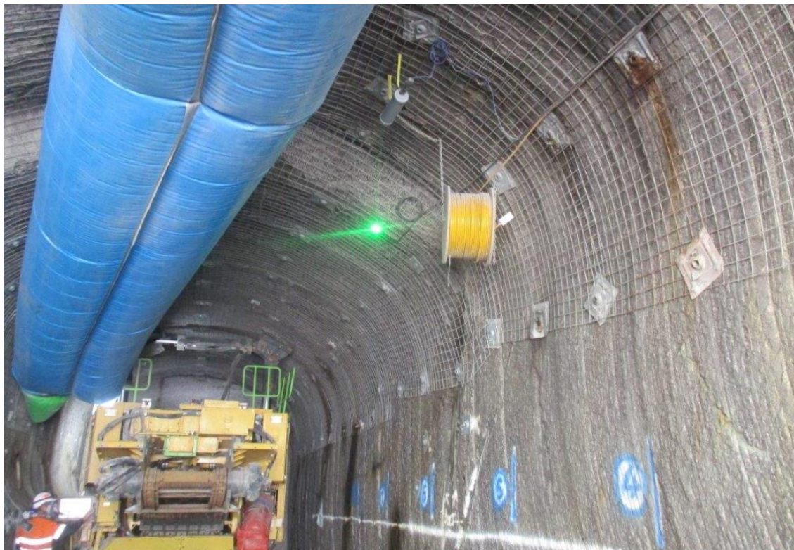
Figure 1 Quality of walls within the decline are exceptional
