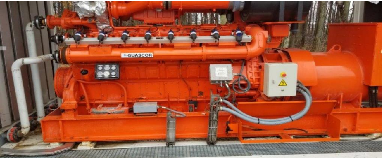
Images 1-4: AXP's Colorado lease ready for the commencement of earthworks (1 & 2) and power generator units being loaded for transportation to site (3 & 4)
