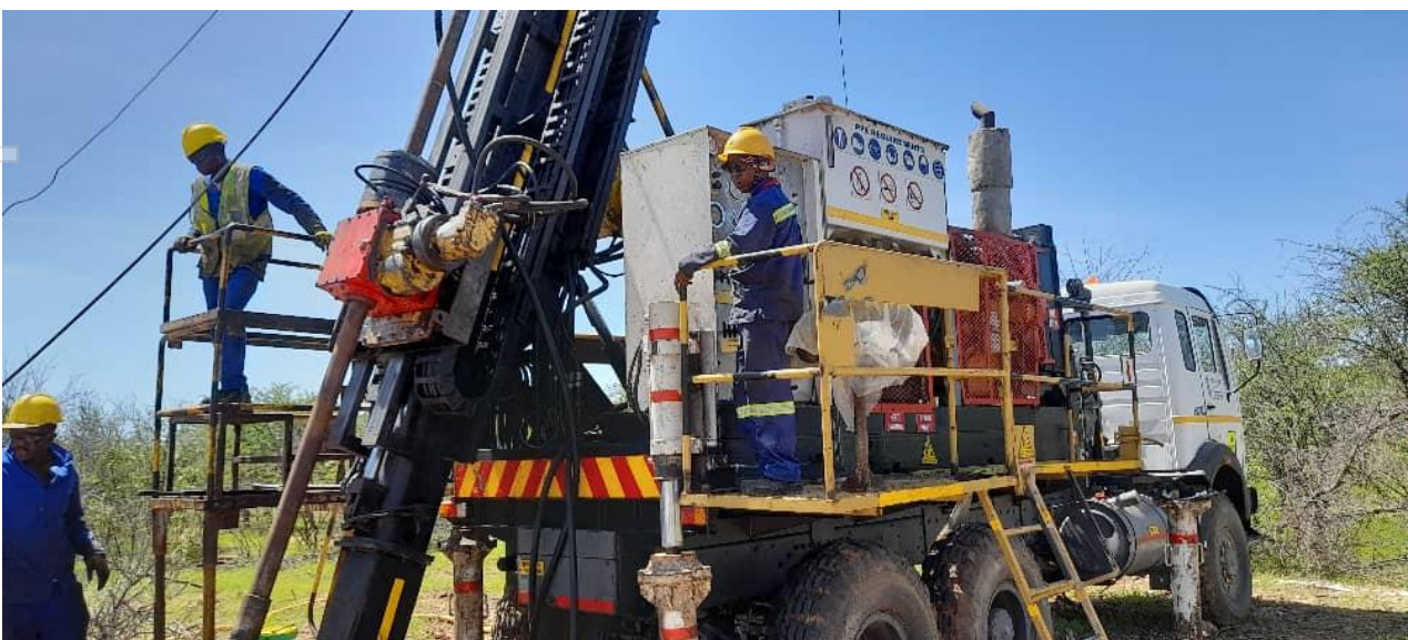
Figure 1: Drilling at Opuwo.
