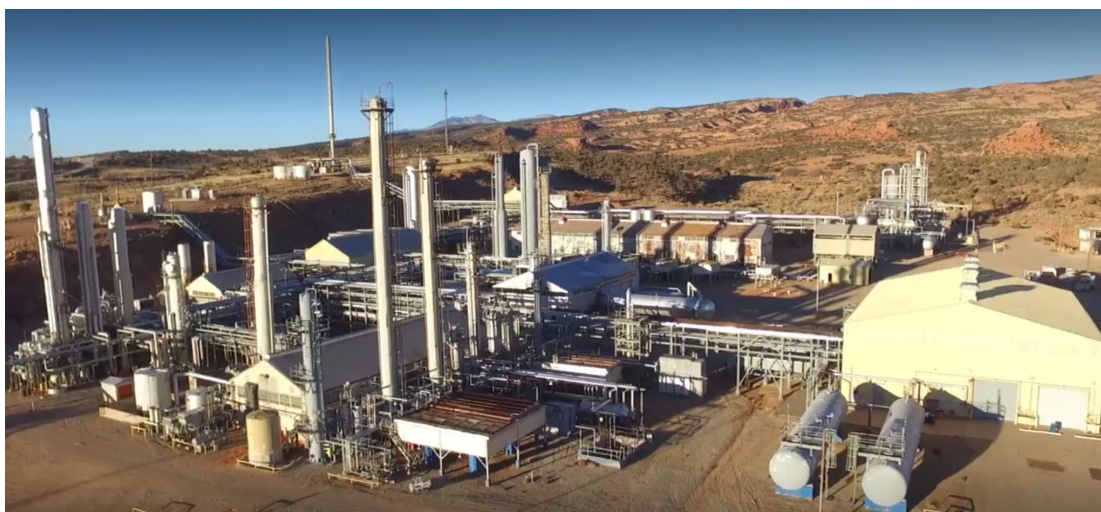
Figure 1: Paradox Resources Lisbon Valley Gas Processing Plant.
