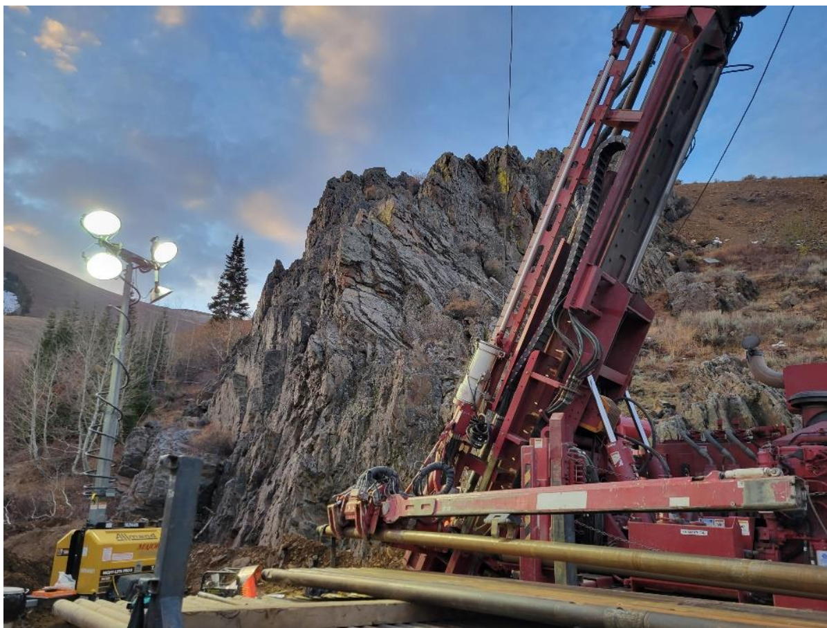
Figure 2: Commencement of RC drilling at Big Springs
