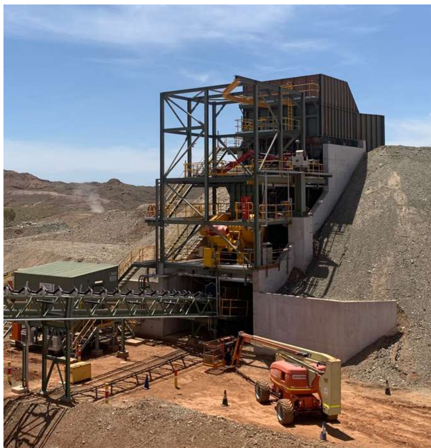
Figure 4: ROM Bin and Crusher
