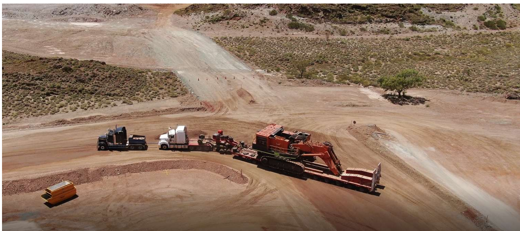
Figure 8: 200t excavator mobilised to Warrawoona
