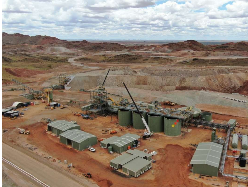
Figure 3: Process Plant Construction – Site View
