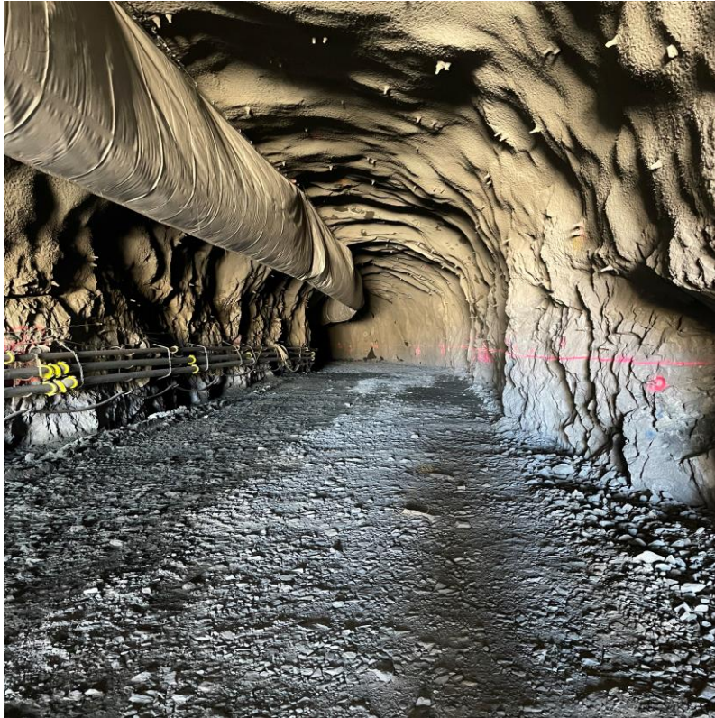
Figure 3: MAT (looking from Portal to first bend)
