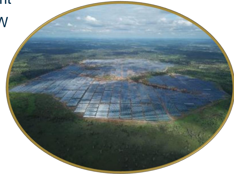
Source: FRV, Photovoltaic Plant, Lilyvale Qld
