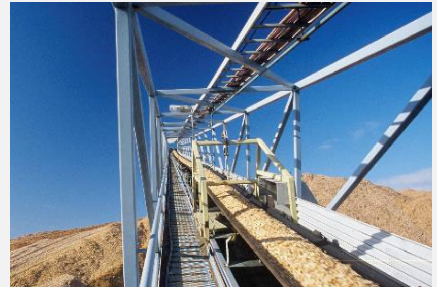
Conveyor health monitoring and intelligence platform
