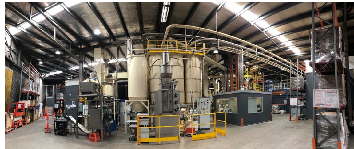
Di Bella Coffee Roasting Facility, Castle Hill, Sydney
