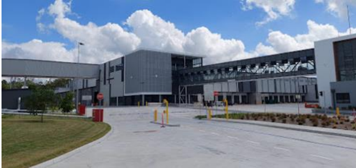
Heathwood Chilled & Frozen DC, Qld New manual chiller and freezer facility Opened ahead of schedule in H1
