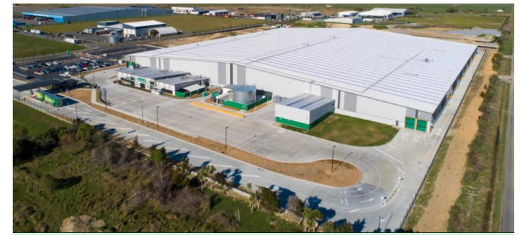
Palmerston North DC, NZ New greenfield ambient DC Opened August 2021
