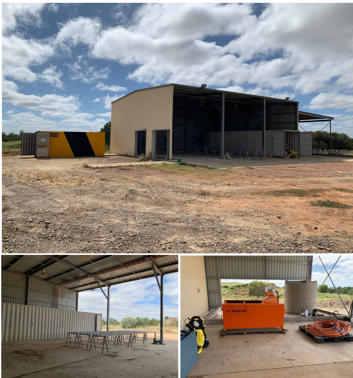
Figure 6: Original mechanical workshop now being re-purposed as dedicated core logging and processing facility. The yellow container is an airconditioned core cutting room that will house a new Corewise™ automatic core saw.
