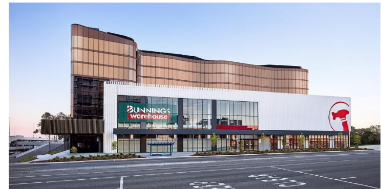
New Doncaster warehouse in Victoria, opened December 2021
