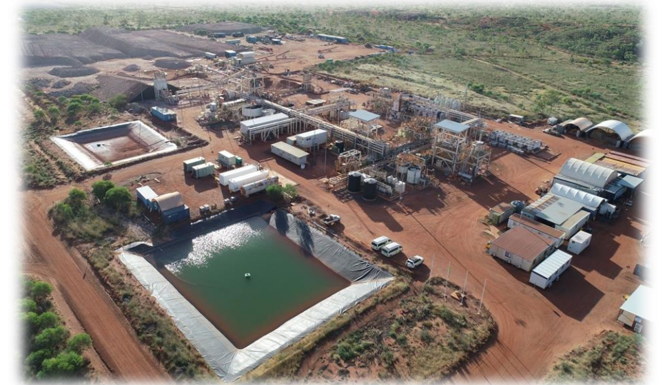
Browns Range Pilot Plant
