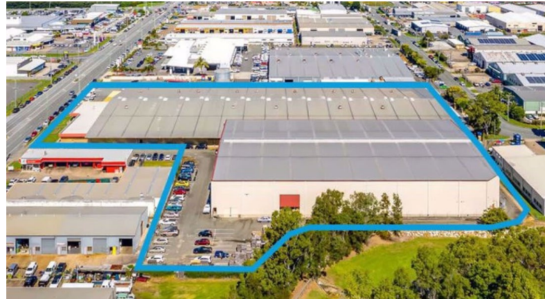
Modern Star Distribution Centre, Brisbane QLD
