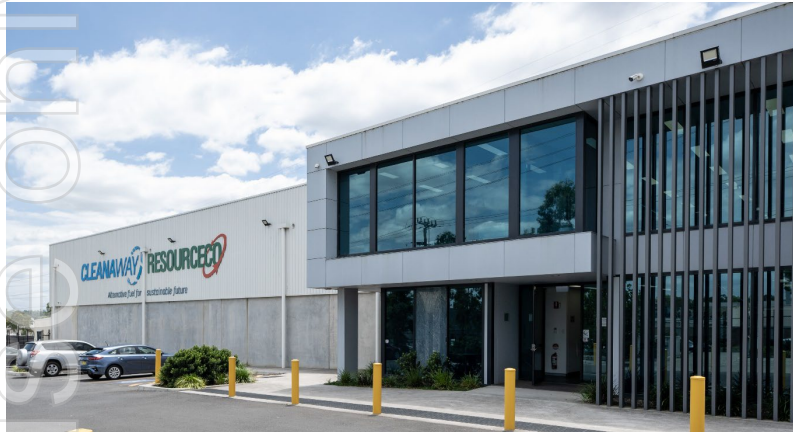
Cleanaway & ResourceCo Facility, Sydney NSW
