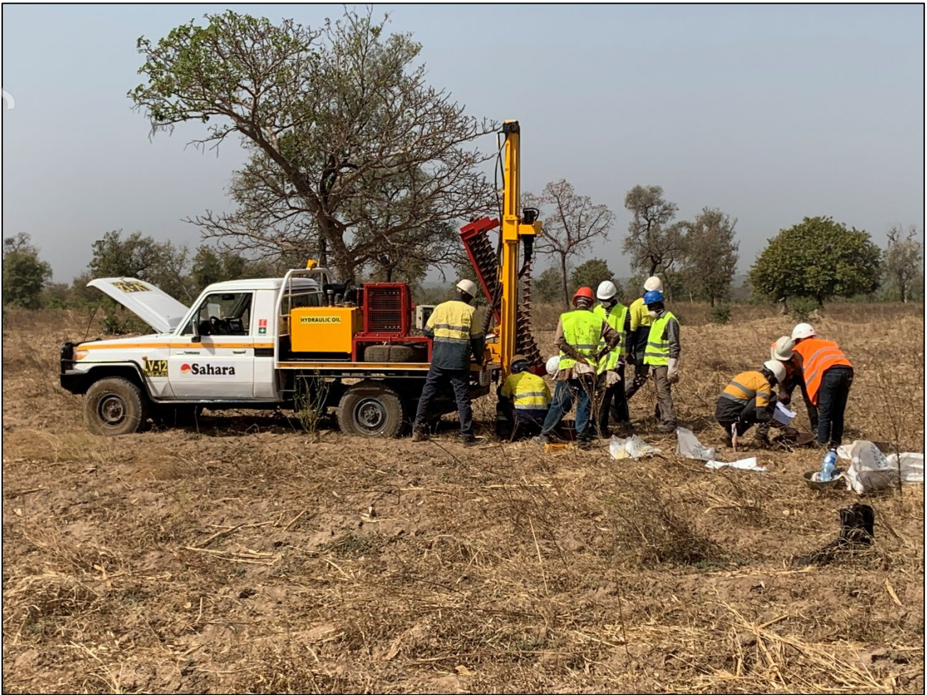
Figure 2: Auger drill on the Korhogo Nord permit
