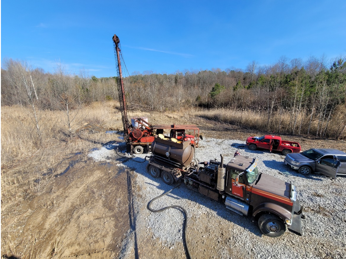
Image 2: Workover underway at DPI-2605 well
