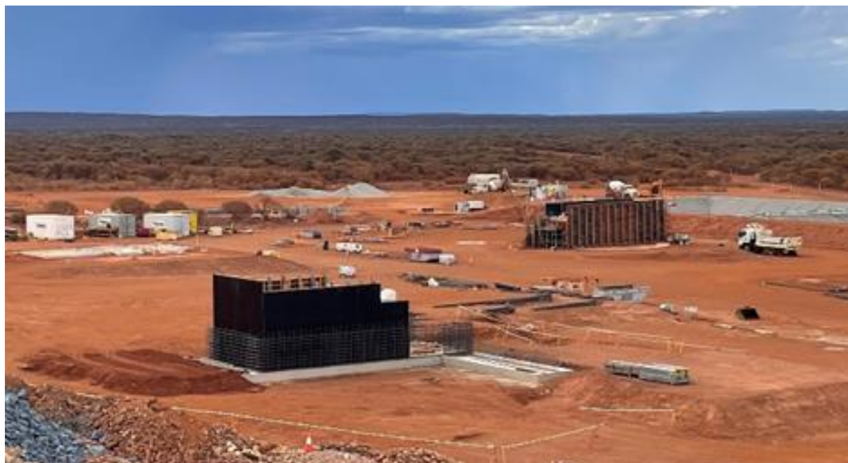
Figure 1 shows some of the Abra processing plant construction activities in January 2022. Concrete foundations being placed in the primary crusher area in the foreground and the fine ore bin (FOB) in the background.
