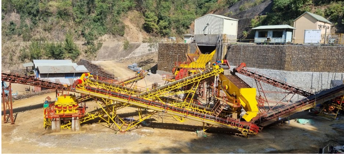
Figure 9. Recommissioned Ban Phuc Crushing Circuit
