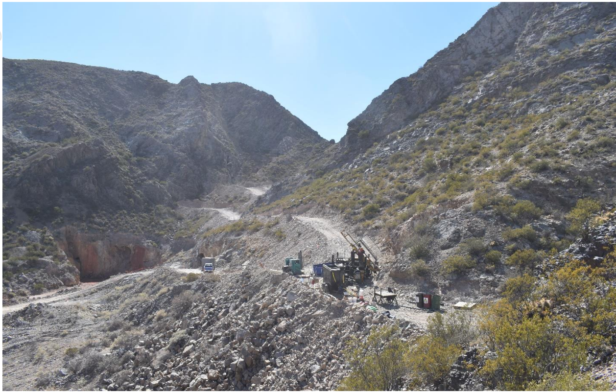
Photo 1 (looking north) - GNDD-397 drilling and road to up-dip drill pads including GNDD-434
