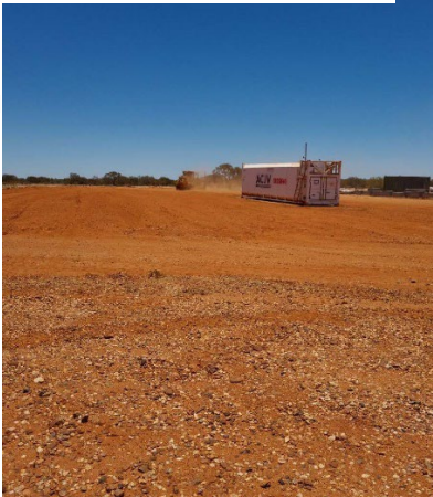
Clearing of the fuel depot area on site
