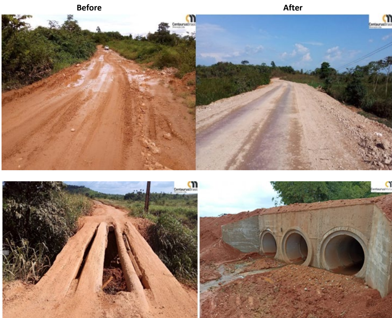
Figure 7 – Road Upgrade Work completed as a result of the Public Private Partnership with the Sao Felix do Xingu Municipality
