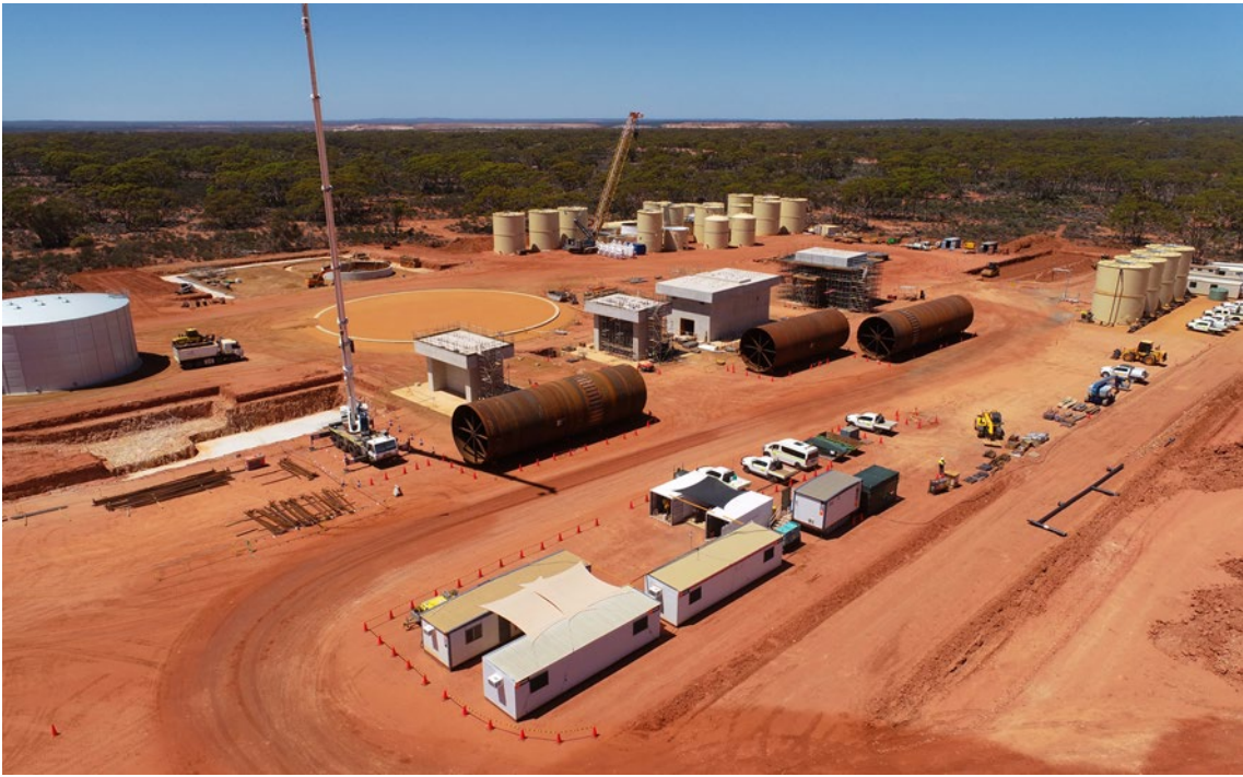
Aerial view of works completed in compliance with minor and preliminary works approval
