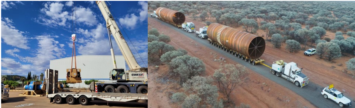
Unloading Kiln Rollers in Kalgoorlie, and kiln shells on their way
