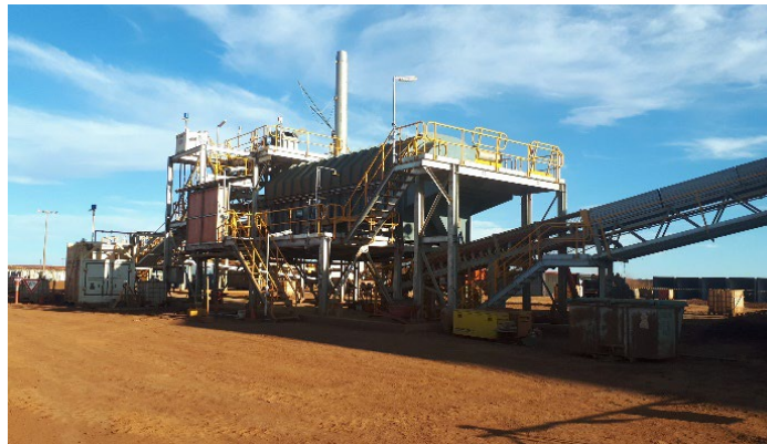
Concentrate Dryer construction completed with pre-commissioning
