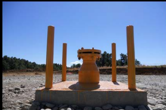
Completed Monitoring Well
