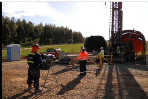
Monitoring Wells - Logging of Well
