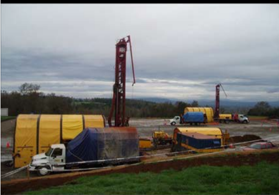
Monitoring Well Drilling on Vertical Drilling Pad
