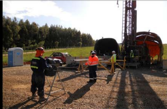
Monitoring Wells - Logging of Well
