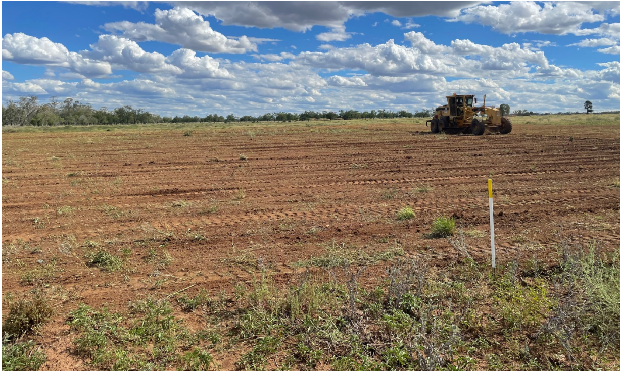
Wellesley-2 Drilling Lease Pegged and Graded
