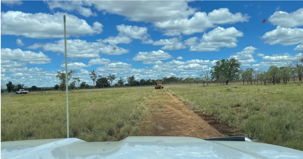
Wellesley-2 Drilling Lease Pegged and Graded
