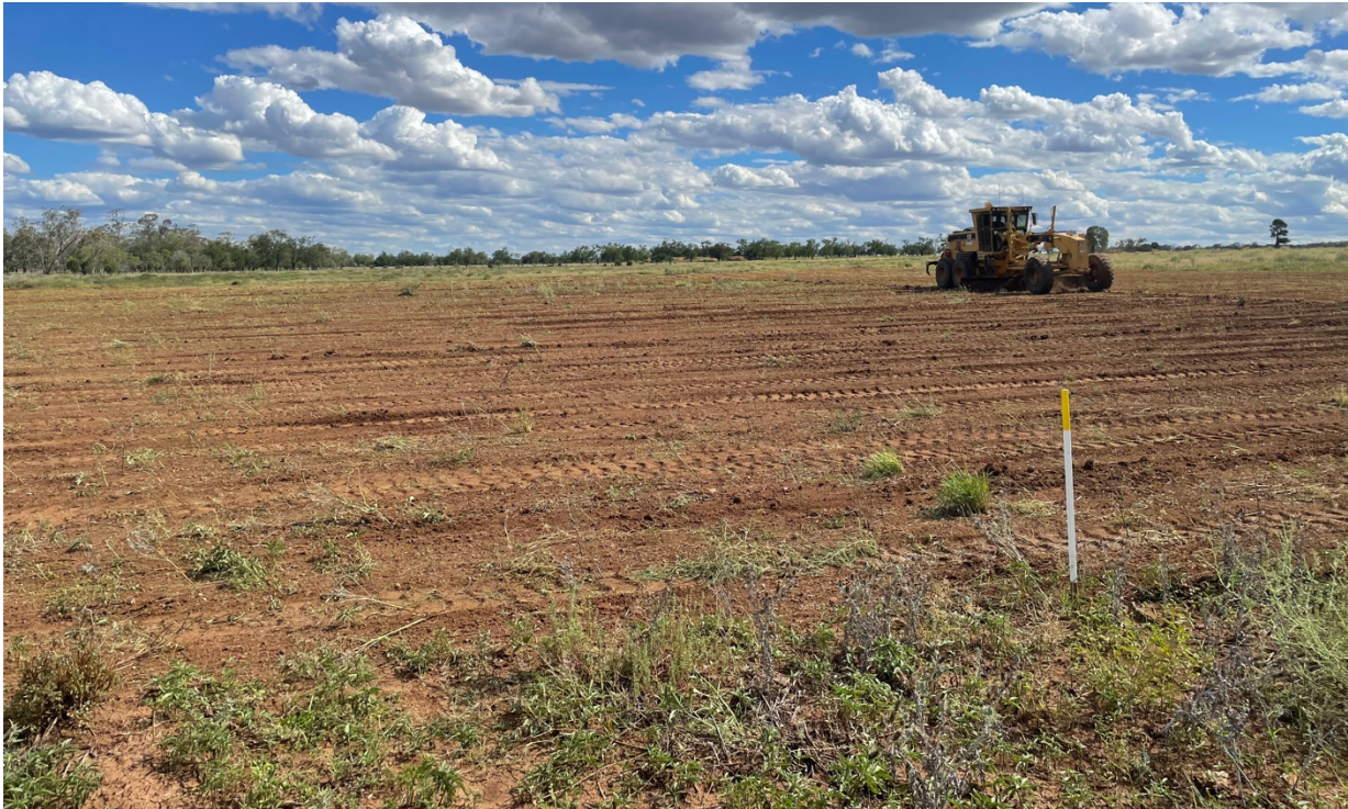
Wellesley-2 Drilling Lease Pegged and Graded
