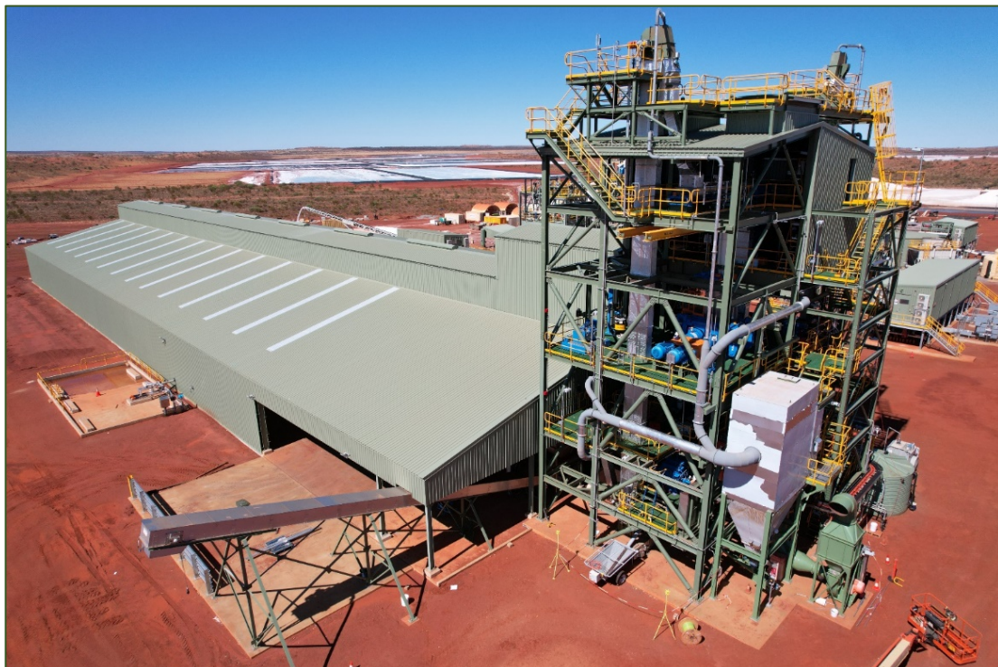
Compaction Plant Construction Complete
