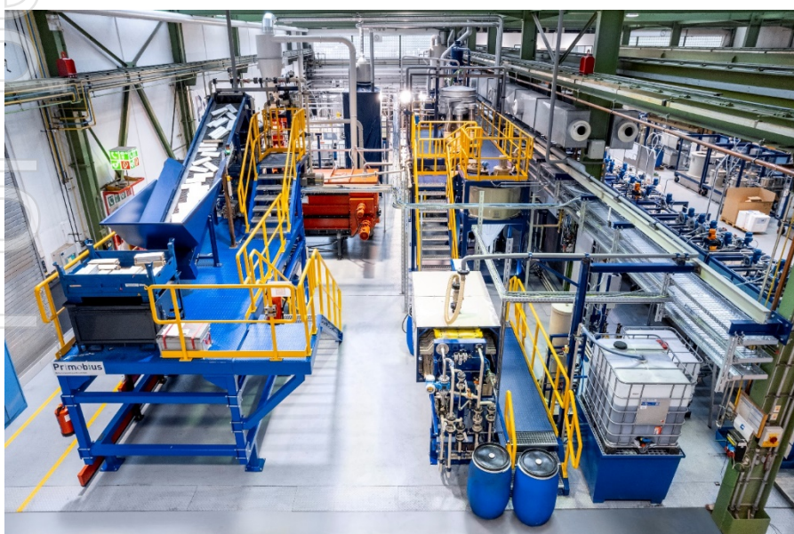
Image 1 - Commissioning with EV cells
