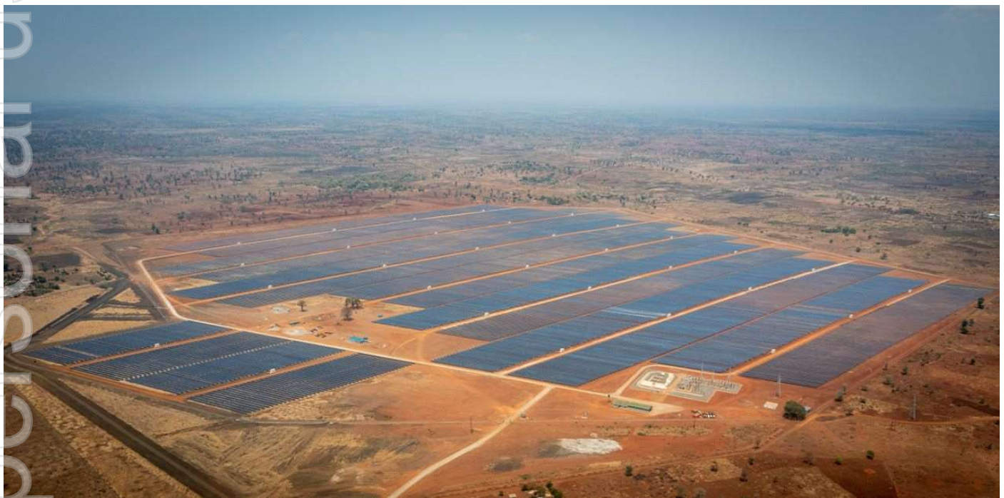
Figure 28: 60MW Salima project in Malawi constructed by JCM (source: JCM)
