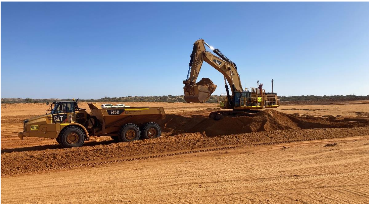
Figure 2 – Ambassador North pit ramp looking north
