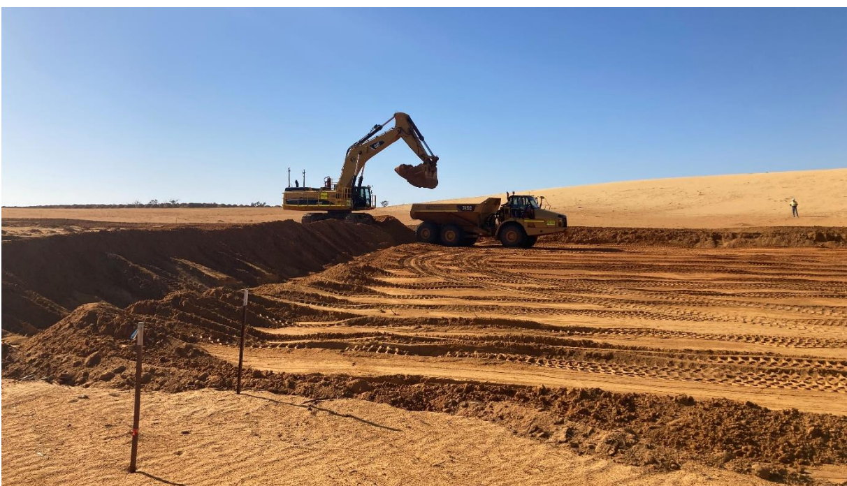
Figure 3 – Ambassador North pit ramp looking south
