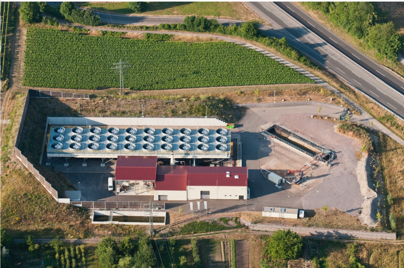
The geothermal power plant in Insheim, Upper Rhine Valley, Germany.
