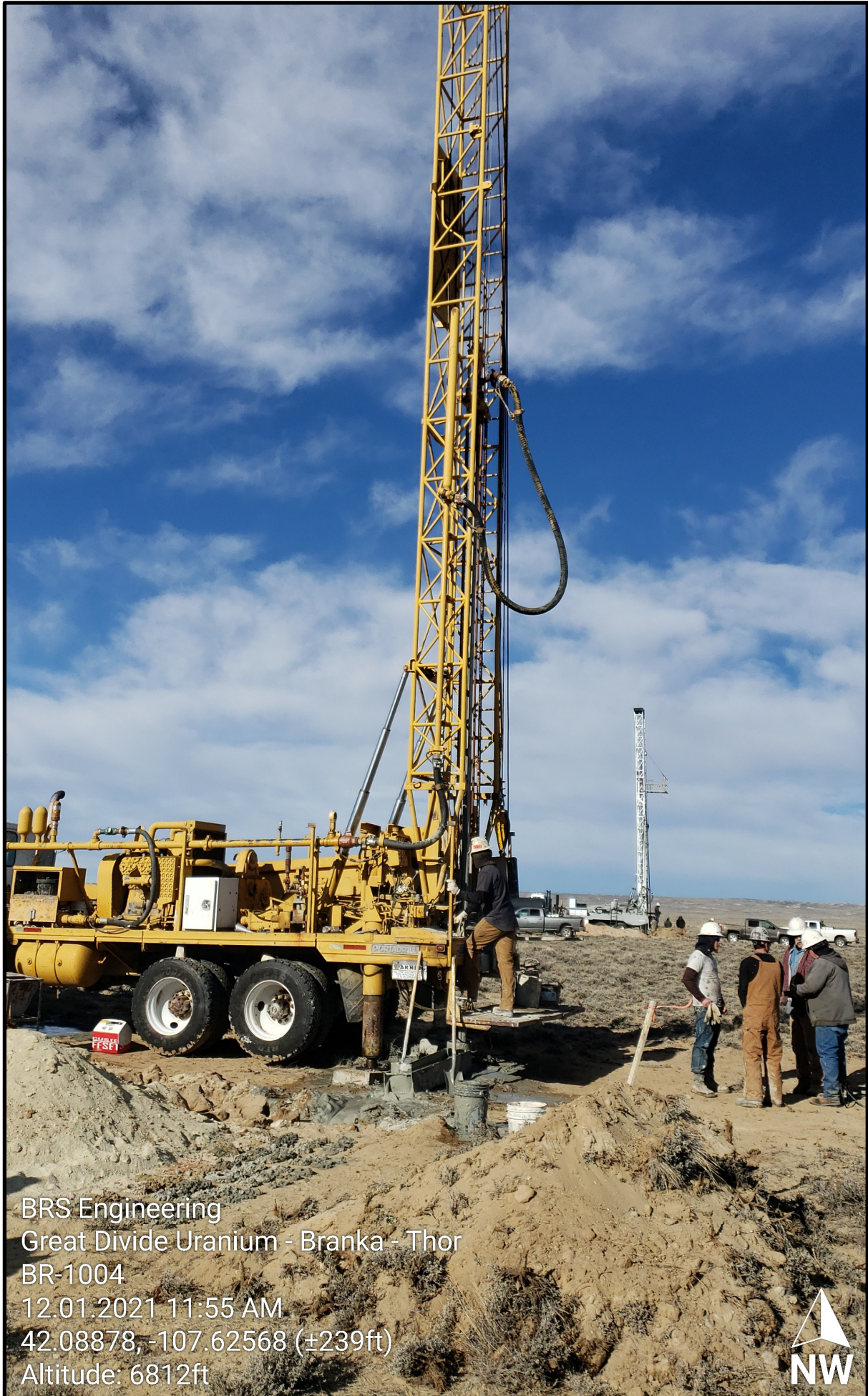
Figure 2. Mud Rotary Drill Rigs (x2), Ancillary Equipment and Support Vehicles at the Thor Project.
