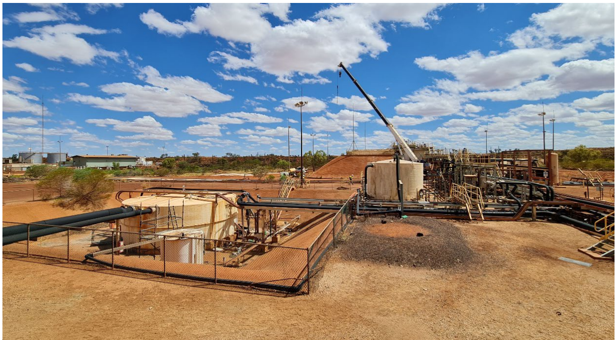
Image 3 / Refurbishment of the Solvent Extraction ("SX") Plant commenced
