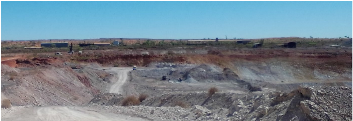
Image 1 / RC Drill Rig on South Eastern end of the Nifty Open Pit
