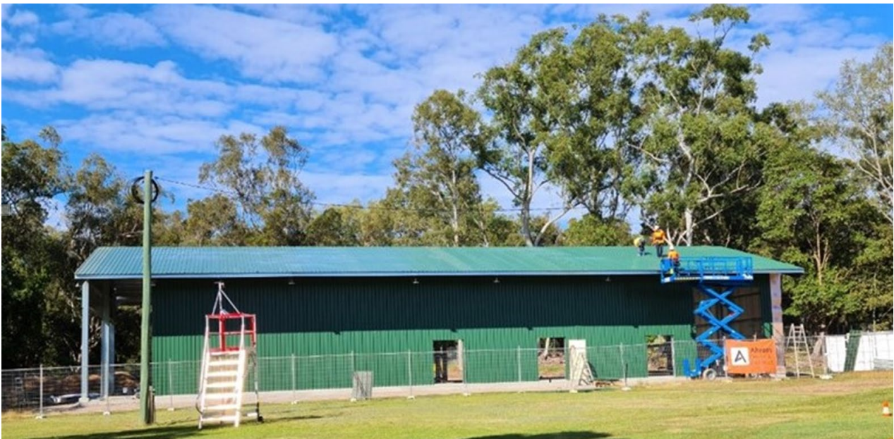
Figure: The Lava Blue research facility under construction in Redlands, Brisbane. The 440 sq m, 6 m high, steel structure will be operating early in 2022 and will conduct repetitive process validation operations, producing 20kg batches of HPA from various materials while developing process control options for commercial scale production.
