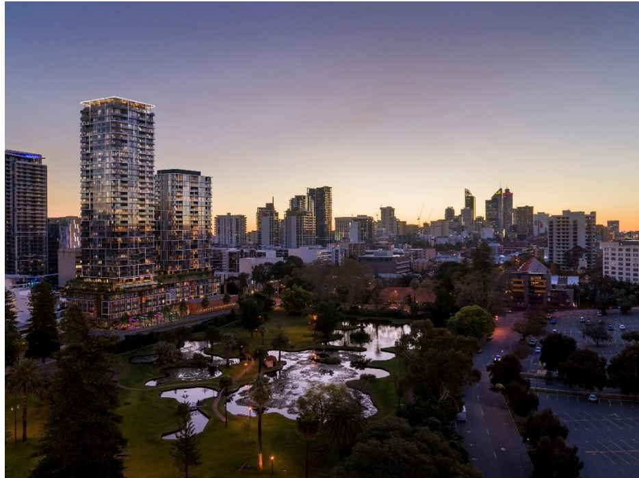
ABOVE: Garden Towers – looking West
