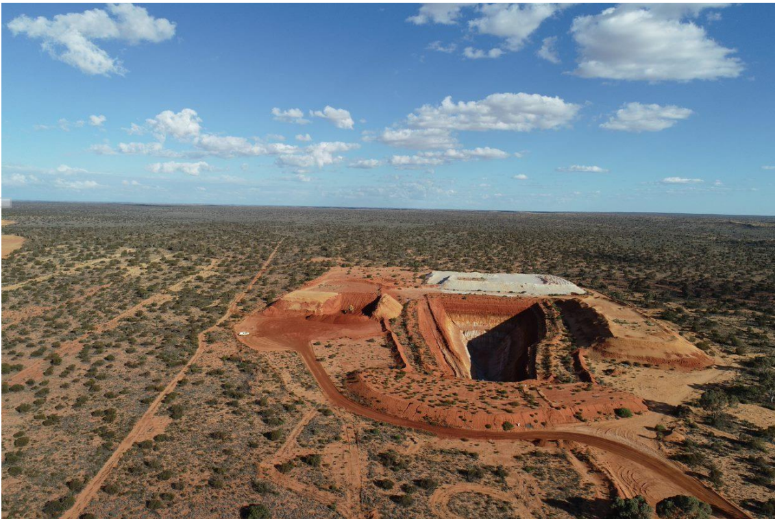
Figure 8 – Ambassador East GIT facing northwest (23 November 2021)
