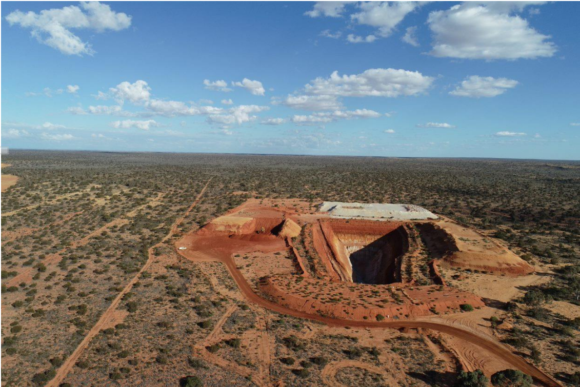
Figure 8 – Ambassador East GIT facing northwest (23 November 2021)
