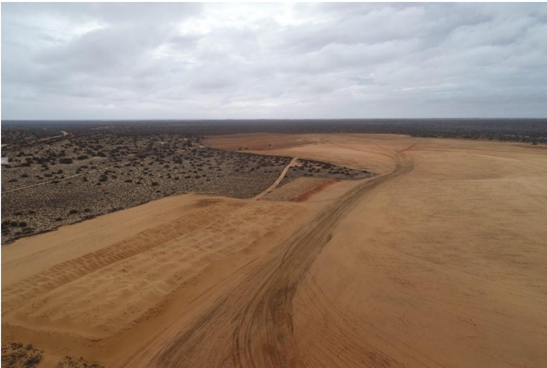
Figure 2 – Topsoil stockpiles at Ambassador North looking east (18 November 2021)
