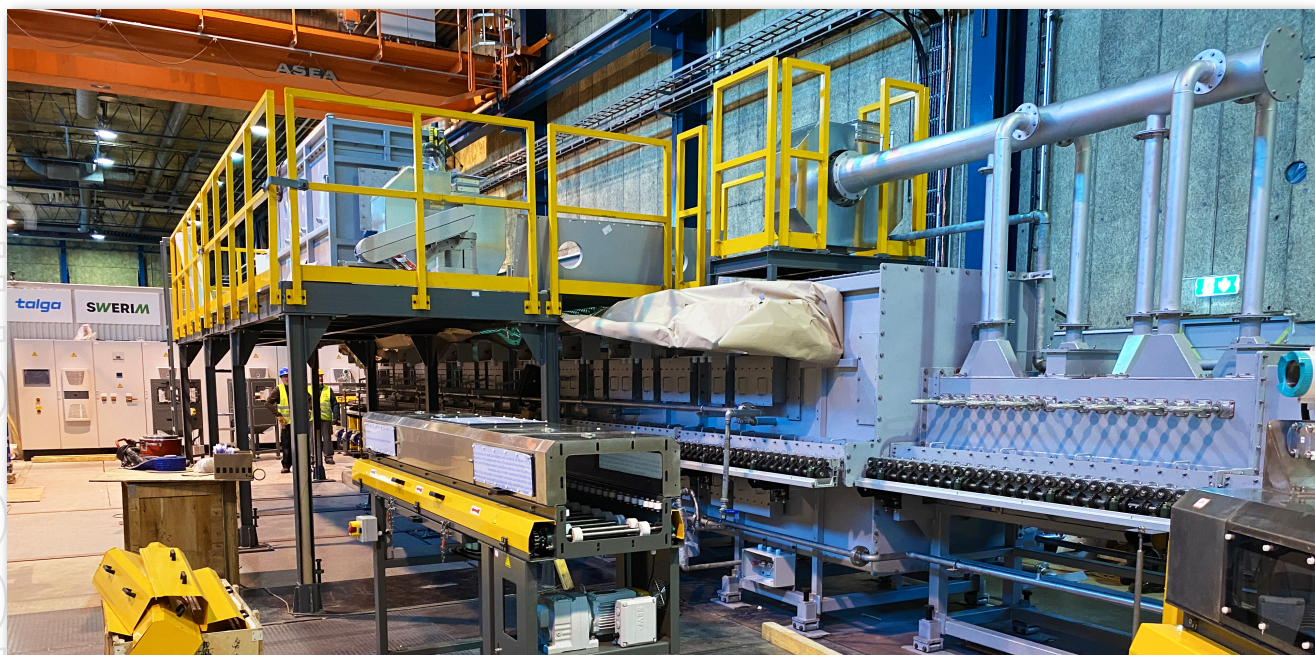
Figure 2 Construction of coating pyrolysis line at Talga's EVA plant in Luleå, Sweden
