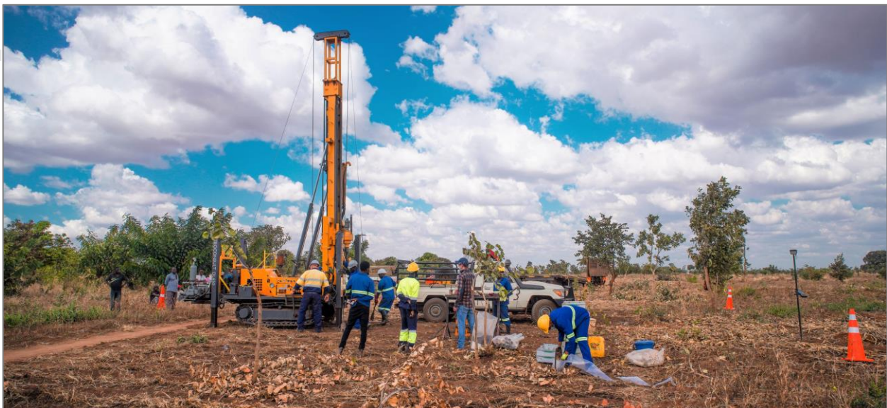
Figure 3: DL650 push-tube core drilling rig in operation at Kasiya
